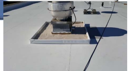
A new grease trap was constructed around a large exhaust unit. The trap was lined with TPO membrane and then filled with sand.
