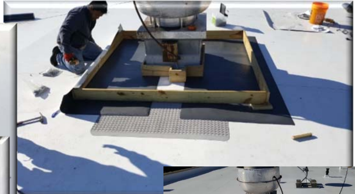
A new grease trap was constructed around a large exhaust unit. The trap was lined with TPO membrane and then filled with sand.
